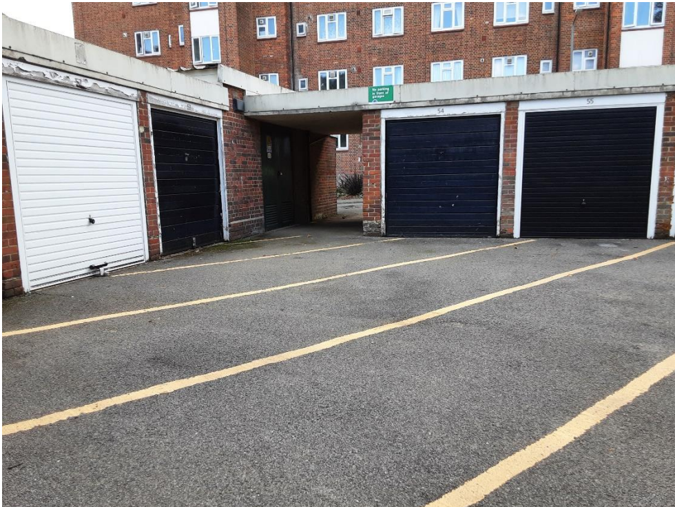
Photograph 4: Example of hardstanding areas and Building 1 on Site 1
